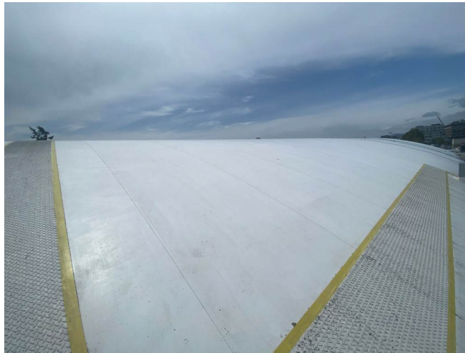
Photo #16: TPO Roofing
