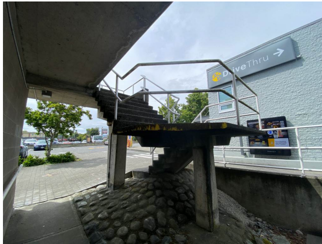
Photo #7: Exterior Concrete Stairase.
