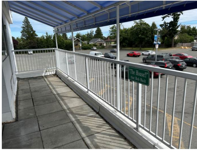
Photo #4: South Balcony
