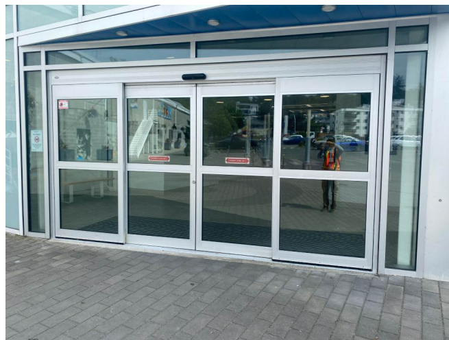
Photo #22: Main Entrance Door
