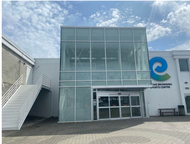
Photo #19: Main Entrance Curtain Wall System
