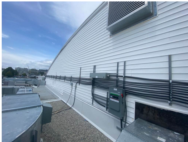
Photo #9: Vinyl Clad Walls
