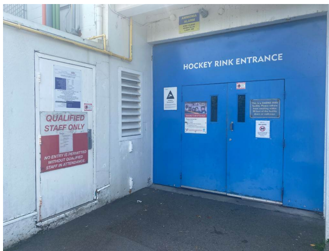
Photo #24: Service Doors, typical
