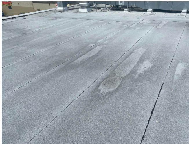
Photo #14: 2-Ply SBS Roofing in Serviceable Condition
