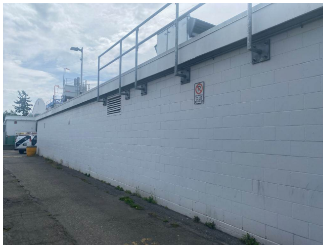
Photo #11: CMU Walls, Painted
