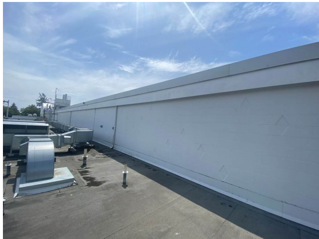
Photo #12: 2-Ply SBS Roofing in Fair Condition
