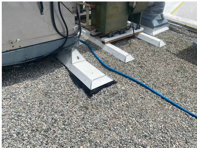
Photo #15: 2-Ply SBS Roofing with Gravel Balast
