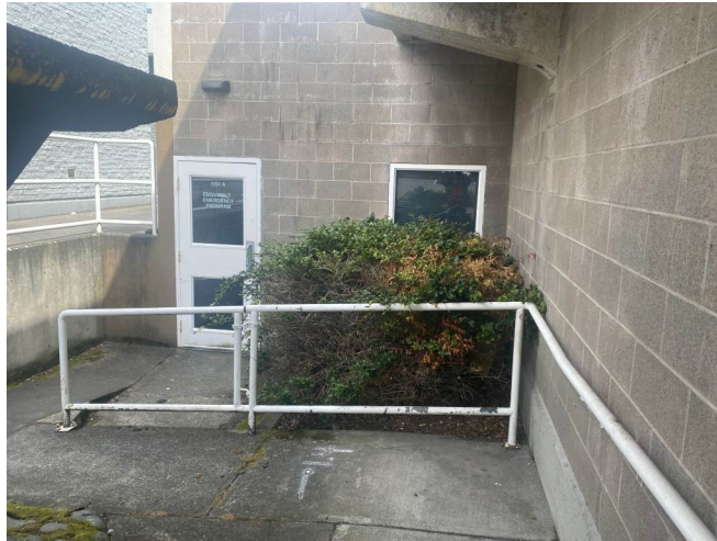
Photo #10: CMU Walls- Unpainted
