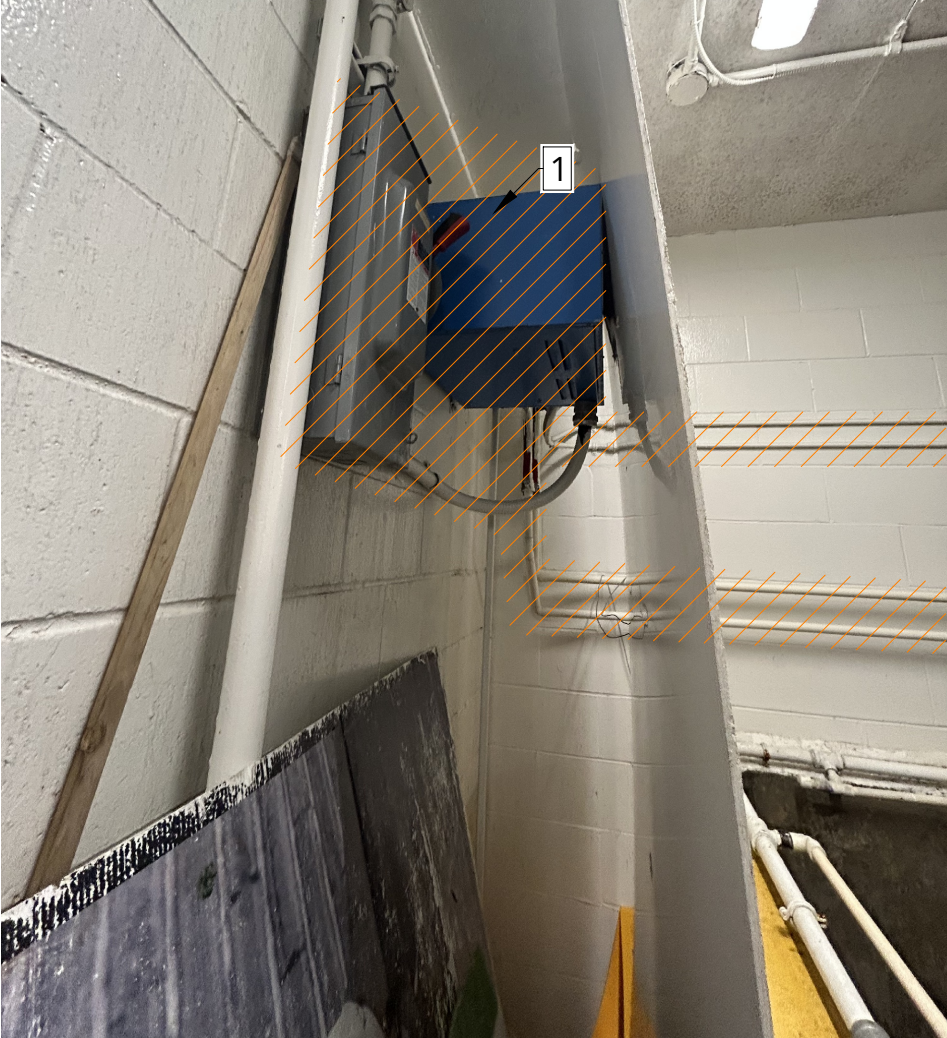
7 SNOW MELT PIT - BOILER DEMO M1 KEYED NOTES: DECOMMISSION AND DEMOLISH ELECTRIC SNOW MELT PIT BOILER AND ADJACENT ELECTRICAL EQUIPMENT. CONTRACTOR TO CONFIRM ELECTRICAL EQUIPMENT WAS CONNECTED SOLELY TO THIS BOILER PRIOR TO REMOVAL.
