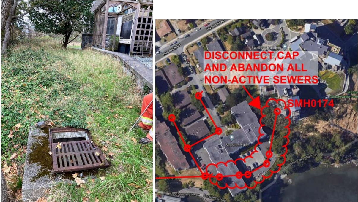
Figure 5-4: Area Draining to Combined Manhole at 847 Dunsmuir Road
