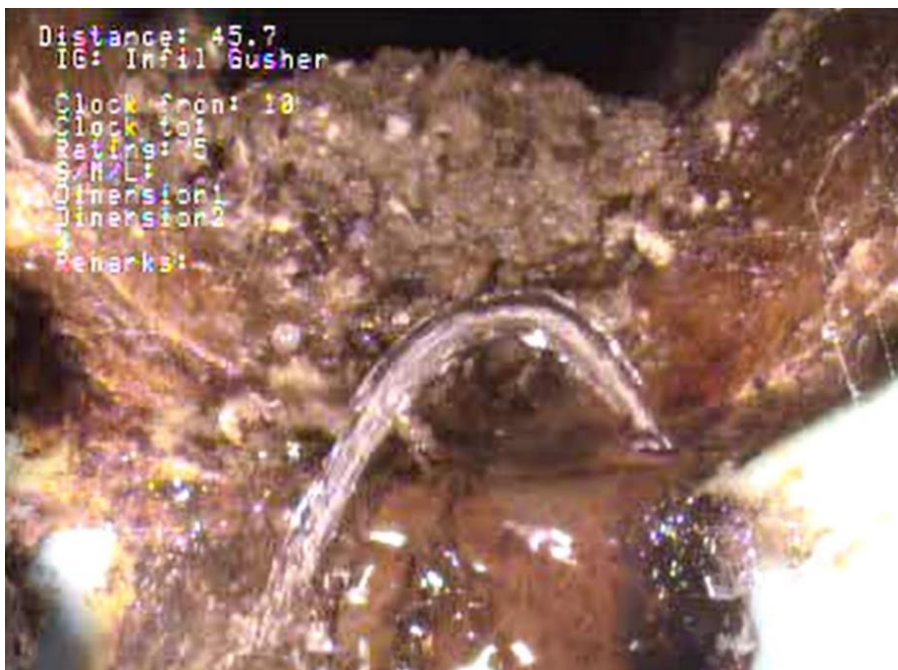
Figure 6-7: I&I at a Lateral Cutout (Picture 2)
