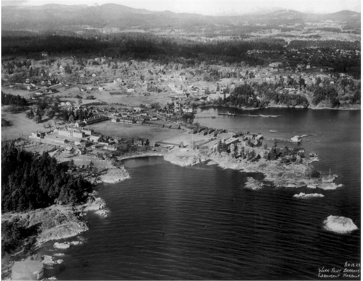
Work Point Barracks [Esquimalt Archives]
